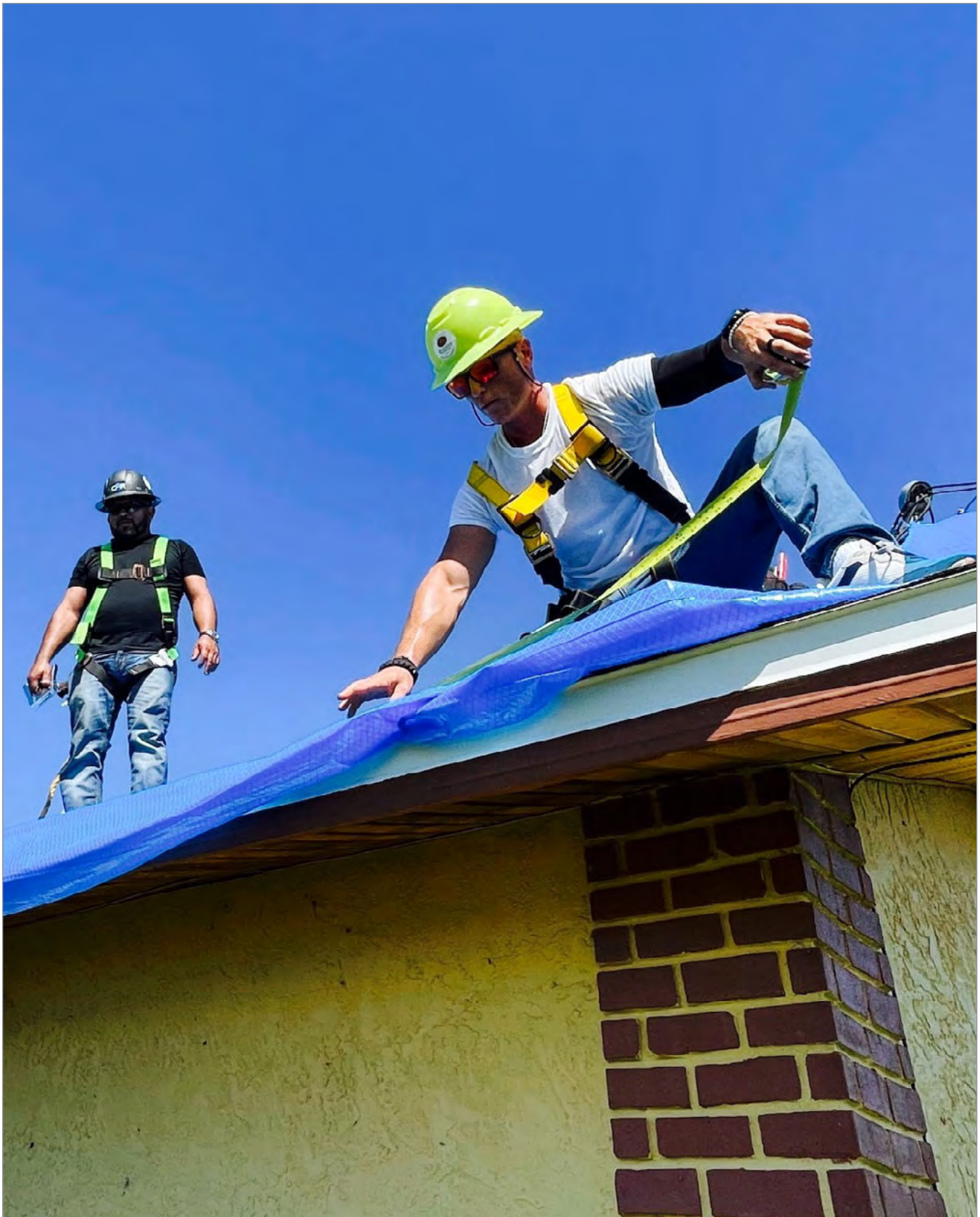
Members of the Army Corps of Engineers install blue, protective sheeting on homes affected by Hurricane Ian in Fort Myers, Florida. Source: Federal Emergency Management Agency.
